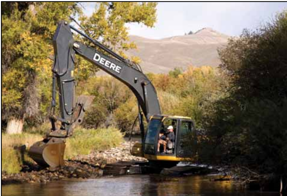
Top: Spring creek as it transitions through a slightly steeper section flanked by willows and cottonwoods. Below: Pulling some of the stream into a designed riffle area and point bar. This area was without a thalweg or suitable fish habitats.
